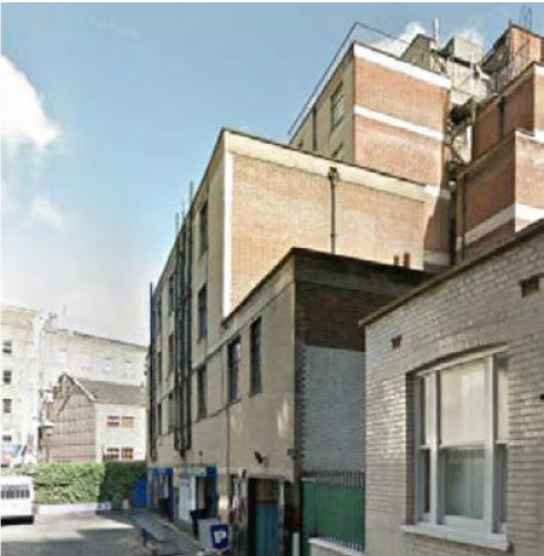
Street view of the south elevation
